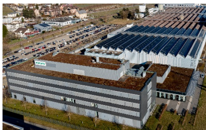
Image 1: The most powerful photovoltaic plant in EKS’s Swiss area is now producing electricity on the roofs of Syntegon at Beringen. It is to be expanded in the years ahead.
