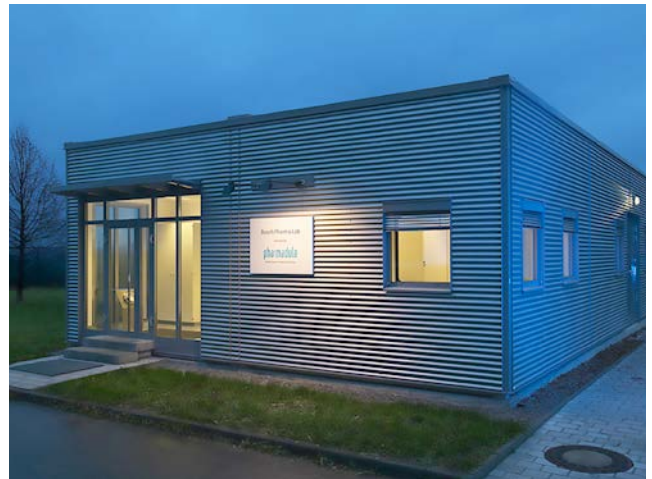
▲ Exterior view Pharmalab Crailsheim
